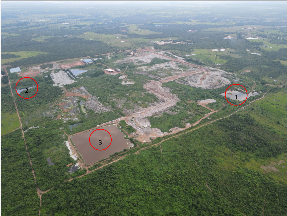
Figure 10 Ponds on the Km 32 Landfill, 06 September 2022
